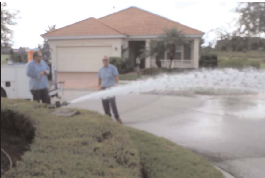
Phil Carnell and Dave Guilmette are flowing a 2 inch meter as part of the quarterly flushing program, which is a requirement by the Department of Health. This program keeps the dead-end water lines located throughout the city from having stagnant water from lack of movement.
