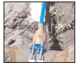
Brandon Dilmore, left, and Jimmy Bennett prepare to replace and repair a 2-inch water service line in the 600 block of South Harbor Drive. Bennett is using the Vactor truck to vacuum the spoil out of the work area, while Dilmore guides it safely around the work area. Lower left, the broken wheel valve and tapping saddle that was leaking through the valve packing. Lower right, the new tapping saddle and corporation stop that replaced the damaged parts. Other employees who assisted are Vadim Bugayev, Marc Richard, Phil Carnell, Jeremy Petrosky, Tony Ramirez, Sal Denato, Marko Tucak, Lee Krauss, Dennis Rodriguez, Carolyn Hart and Stacy Mckenzie.
