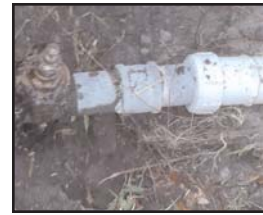
Brandon Dilmore, left, and Jimmy Bennett prepare to replace and repair a 2-inch water service line in the 600 block of South Harbor Drive. Bennett is using the Vactor truck to vacuum the spoil out of the work area, while Dilmore guides it safely around the work area. Lower left, the broken wheel valve and tapping saddle that was leaking through the valve packing. Lower right, the new tapping saddle and corporation stop that replaced the damaged parts. Other employees who assisted are Vadim Bugayev, Marc Richard, Phil Carnell, Jeremy Petrosky, Tony Ramirez, Sal Denato, Marko Tucak, Lee Krauss, Dennis Rodriguez, Carolyn Hart and Stacy Mckenzie.
